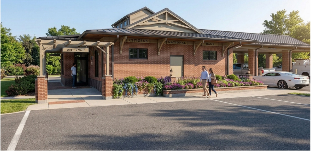
Figure 9: Entry Arbor – West elevation from parking lot.
