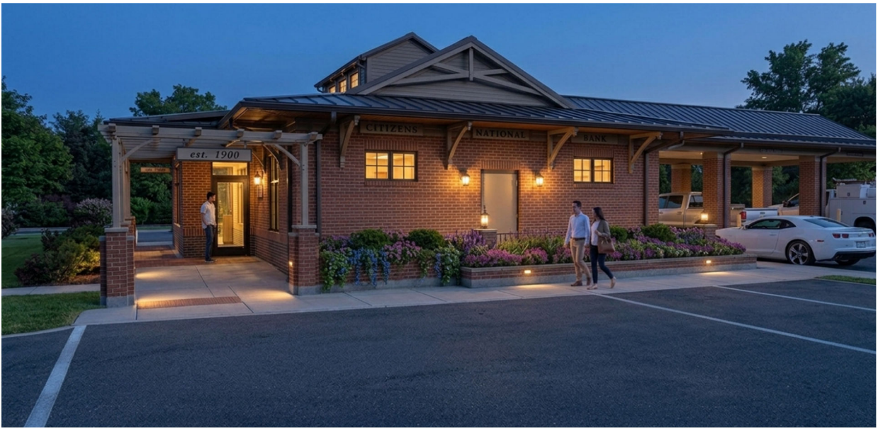
Figure 10: Night View - Entry Arbor – West elevation from parking lot.
